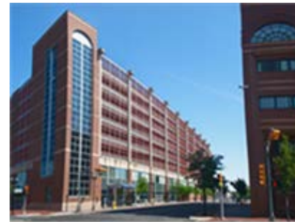
Camden County Technology Center (CTC) – Camden Campus
